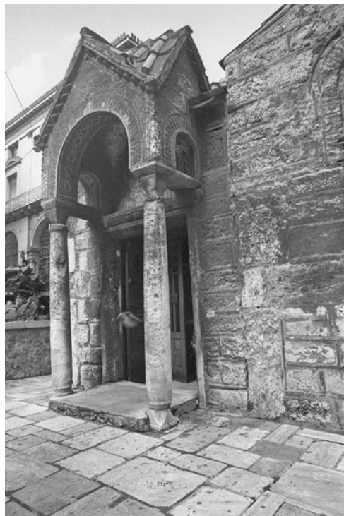
Figure 174 Kapnikarea. The propylon of the exonarthex. View from the southeast.
